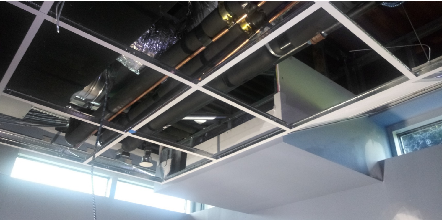
Dispatch 120 – Condensing lines continues at drywall soffit.
