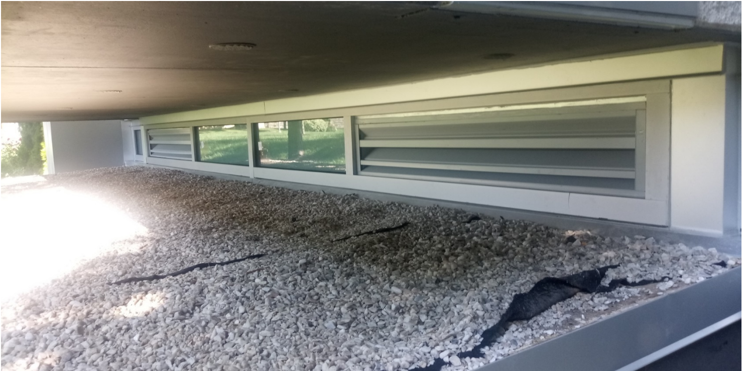
North Elev. – Ballistic window & installations continue.
