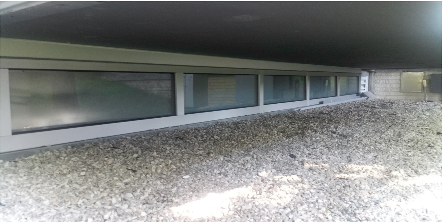
North Elev. – Ballistic window installations continue.
