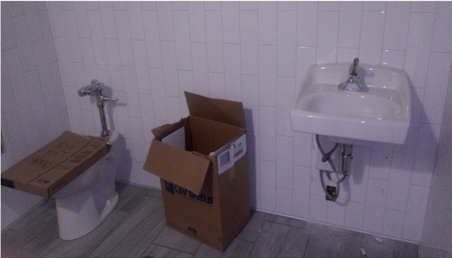
WMN 115 – Plumbing fixture installations continues.
