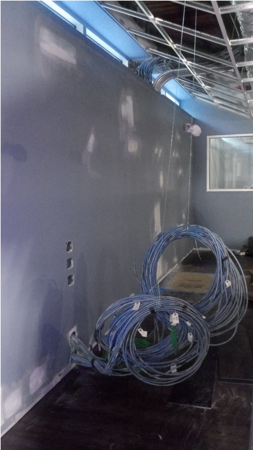
Dispatch 120 – Electrical wiring for Workstations / LVT Installed.
