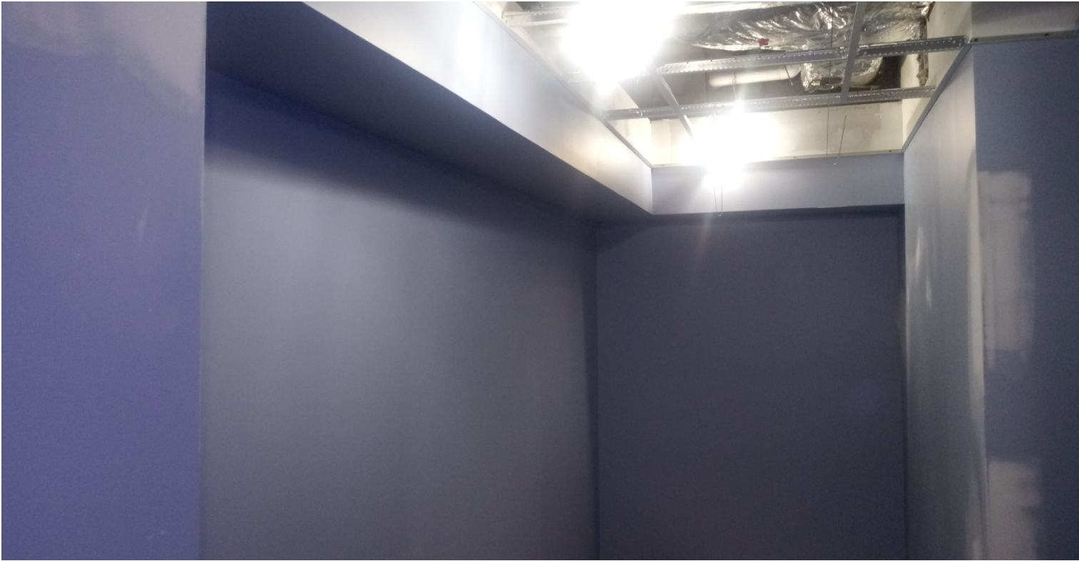
Corr. 118 – Painting continues.
