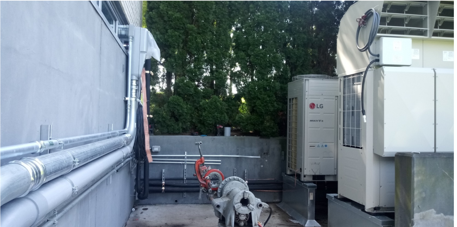
West Elevation – VRF-1 & VRF-2, platforms, & refrigerant piping installation continues.
