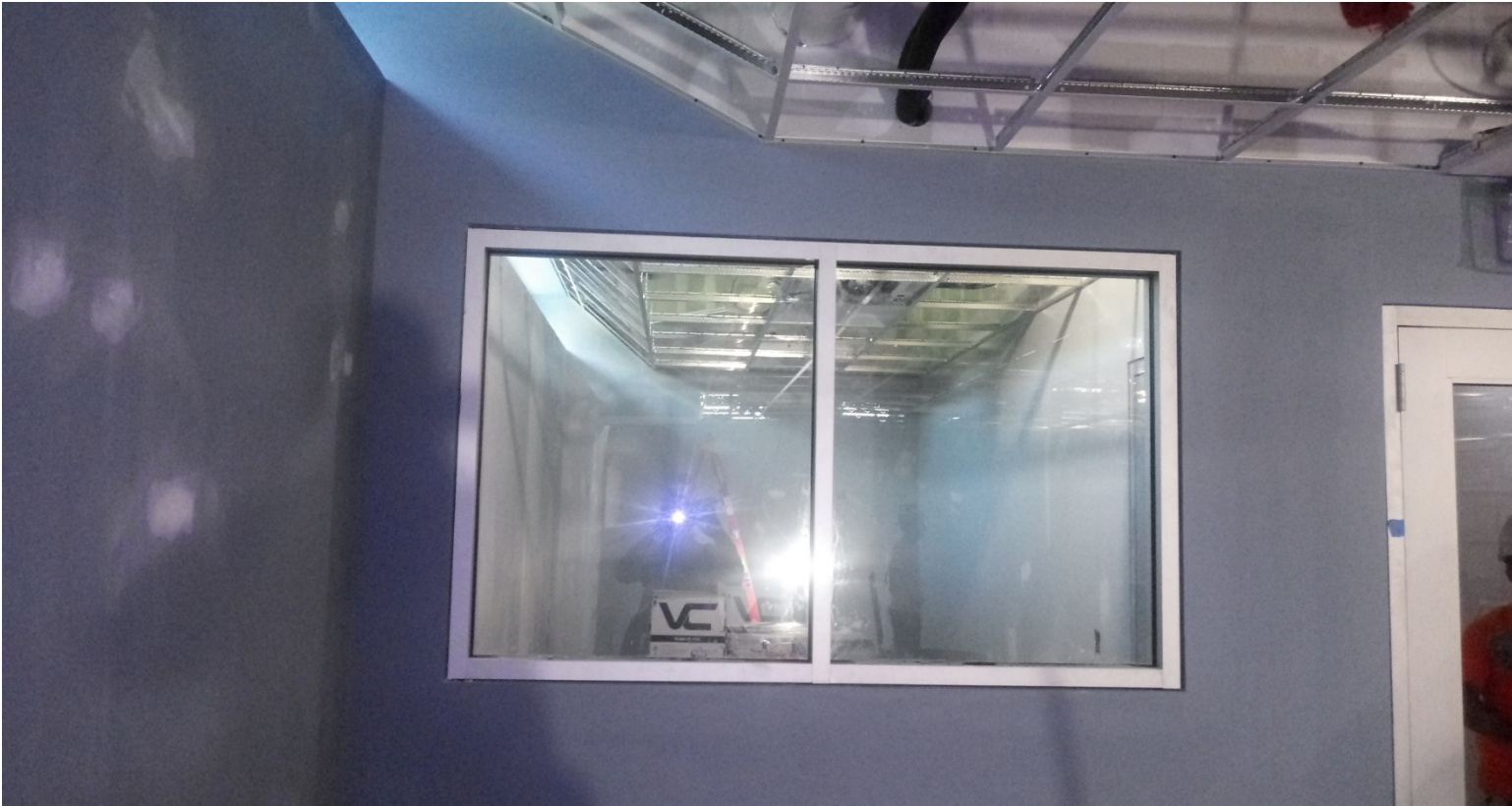
Office 111 – Interior storefront installed.
