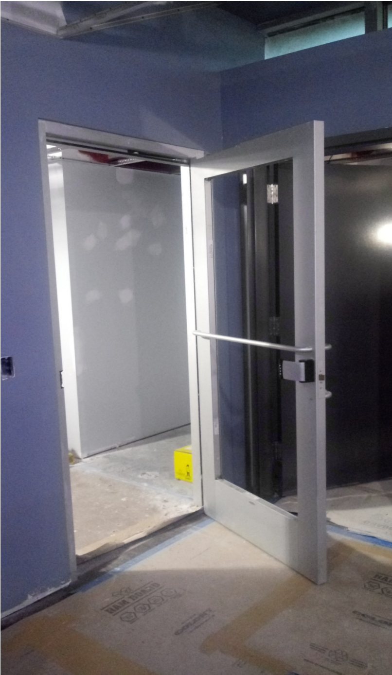
Server Room 122 – Storefront door installation continues.
