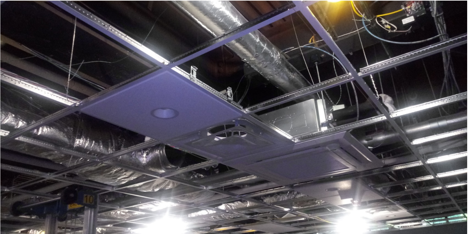
Dispatch 120 – Cassette, Diffuser, & Light fixture installed,
